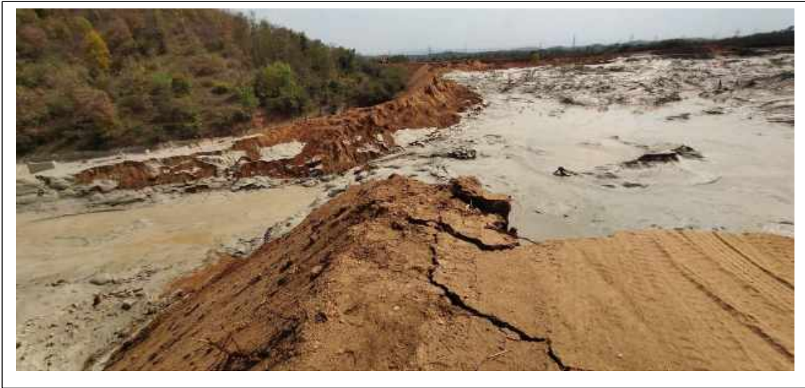
Photograph of the breached site taken on 12.4.2020
