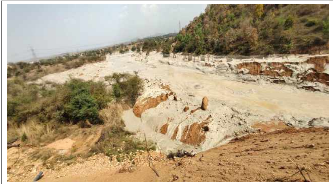
Photograph of the breached site taken on 12.4.2020
