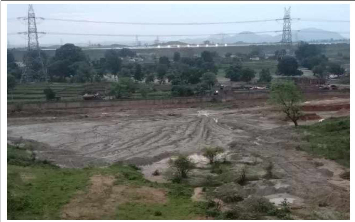
Collected fly ash slurry from Island 4/ C5 area and Goiwahai drain is disposed in low lying area near the Ash dyke 1 & 2 and Island 3 (low lying area)
